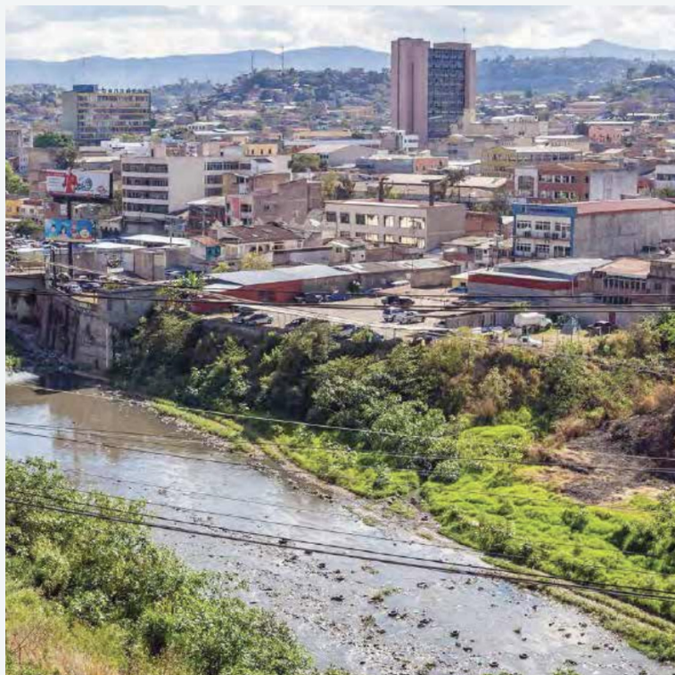
Figure No. 19: Rio Choluteca before the intervention
