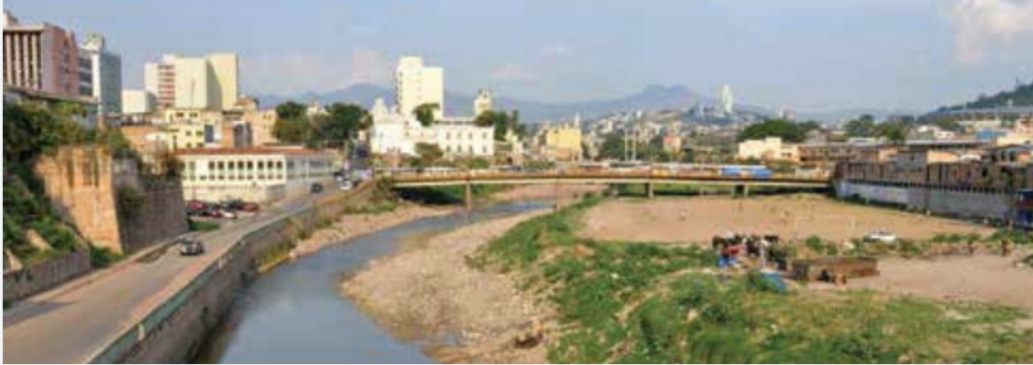
Figure No. 21: Rio Choluteca before the intervention
