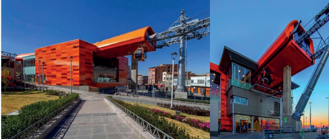
Figure No. 6: Cable Car in La Paz, Bolivia, Substations
