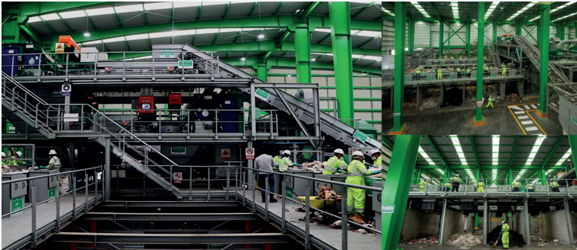
Figure No. 11: Transfer Station and Selection Plant Azcapotzalco, México
