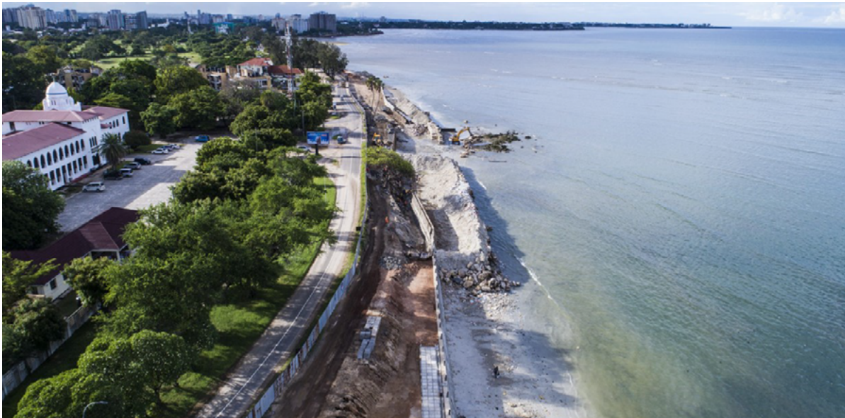
More than 2,400 metres of sea walls were constructed along Tanzania's coast. © UNOPS
