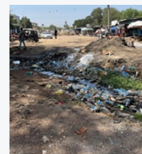
Juba: A small stream carrying wastewater and solid waste crosses the road. Vehicles are forced to navigate through unsafe water, which also poses health risks to people and animals.
